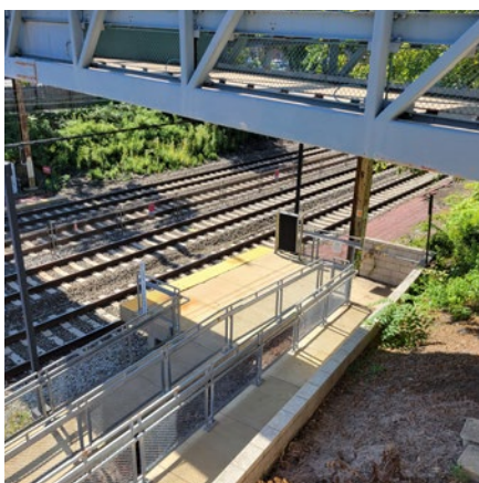
Mini high-level platform at Berwyn meets ADA requirements, but does not confer the other advantages of full-length high-level platforms
