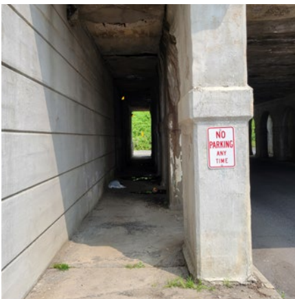
Poor lighting at Coatesville station
