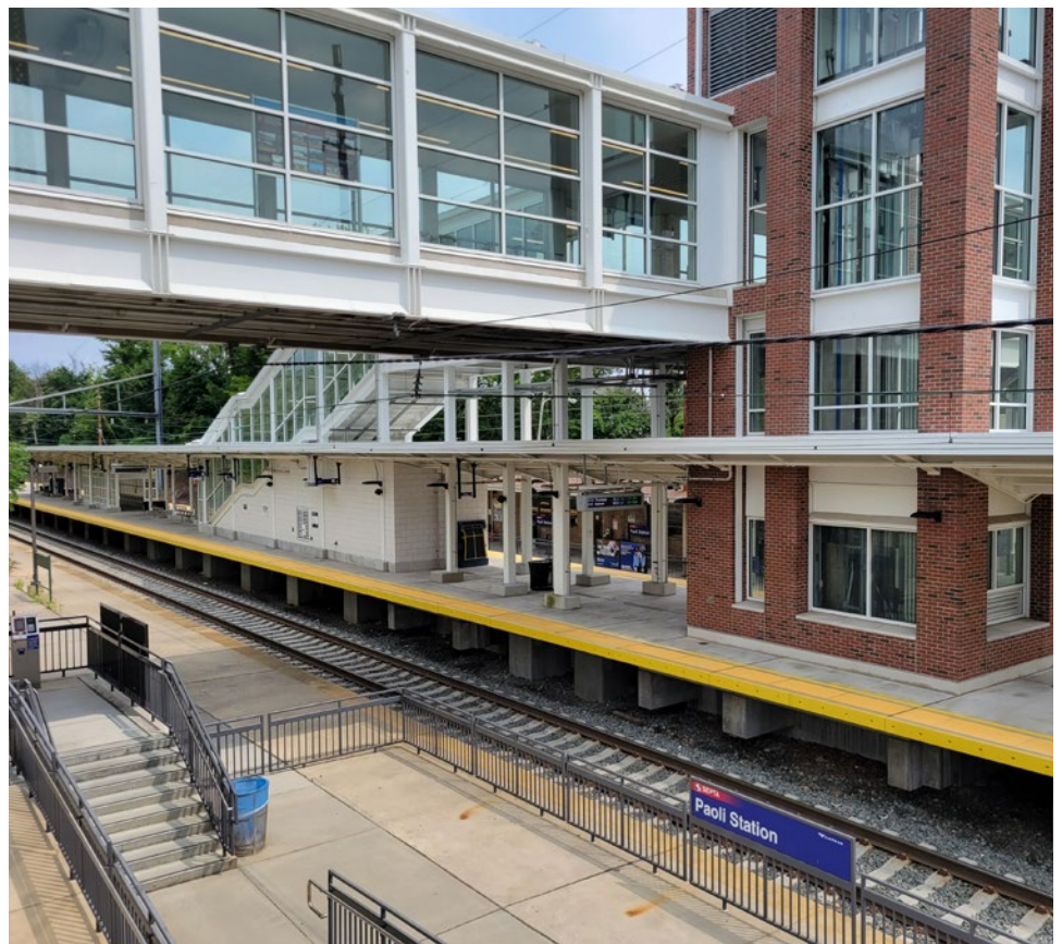
New center island platform and elevators at Paoli
