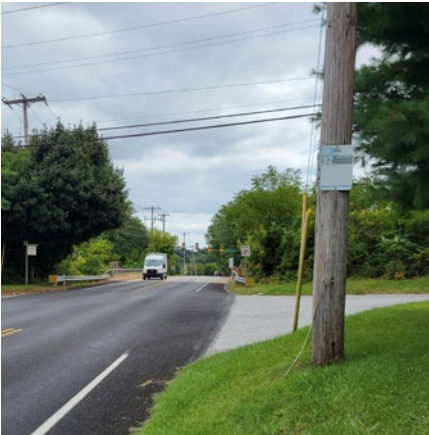
Paired bus stop lacking proper connection
