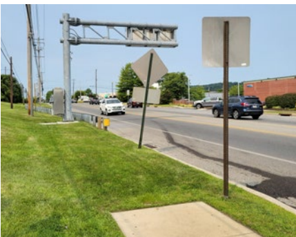
Inadequate pedestrian connections, Thorndale station and adjacent bus stop
