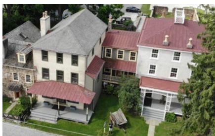
Historic property in Sugartown, Willistown Township.
