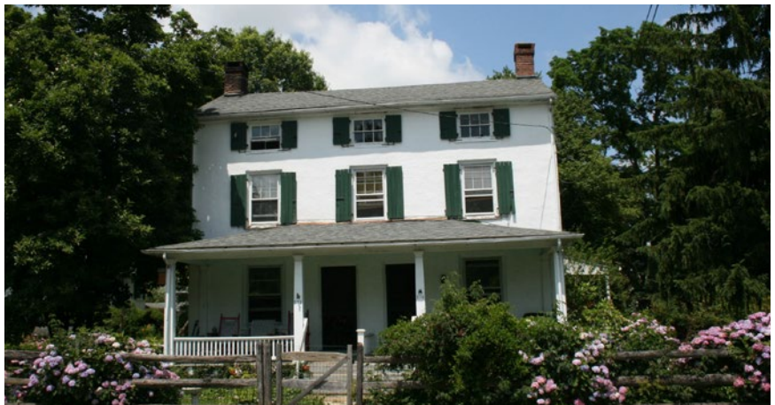
Historic property in Sugartown, Willistown Township
