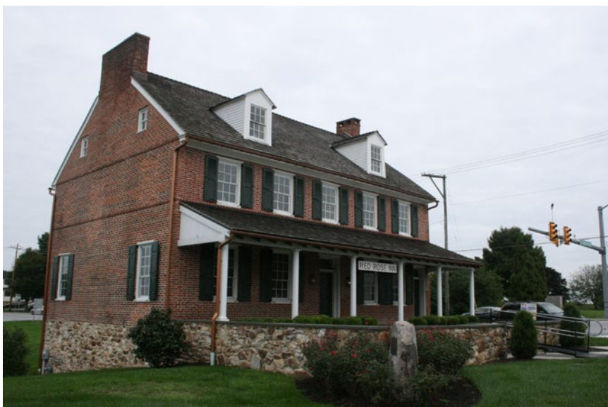
The Red Rose Inn was purchased and rehabilitated by Penn Township.
