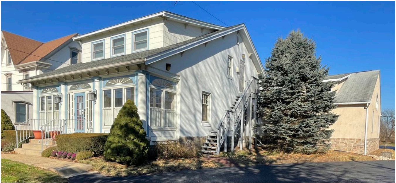
Building addition to the rear of the Pillars of Light and Love property in Trappe Borough, Montgomery County.
