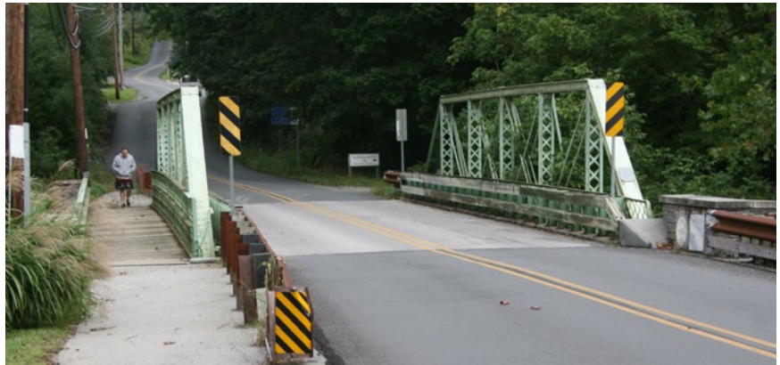
The Landenberg Bridge is an 1899 truss bridge carrying Landenberg Road across White Clay Creek in Landenberg, New Garden Township.
