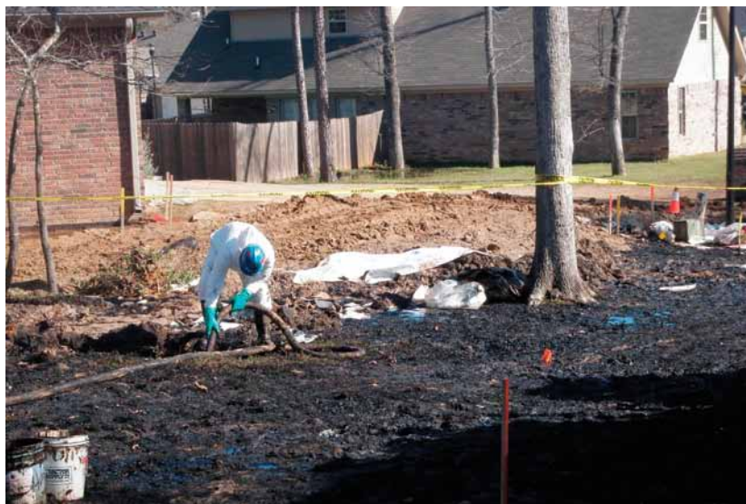
In March 2013, the Pegasus pipeline spilled an estimated 210,000 gallons of heavy Canadian crude oil into a neighborhood in Mayflower, Arkansas. The rupture in the pipeline was caused by cracking along an Electric Resistance Welded (ERW) seam that went undetected by Exxon. (photo courtesy of EPA)
