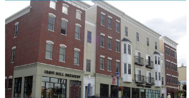
Ground floor commercial space in multi-story buildings
